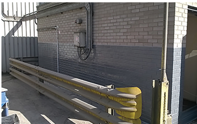
Figure A5.4 Waterproof coating to 1.5 m height applied to external control room walls (courtesy Adler & Allen)
