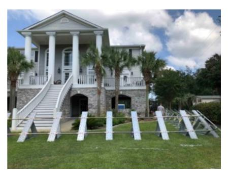
The barriers consisted of a combination of EUR125 Steel Barrier, EUR125 Board Barrier and EUR101 Steel Barrier, side by side – deployed on grass and concrete.
